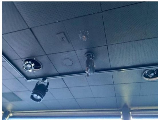
Figure I-5 Damage Within Existing ATCT Due to Leaking Roof
