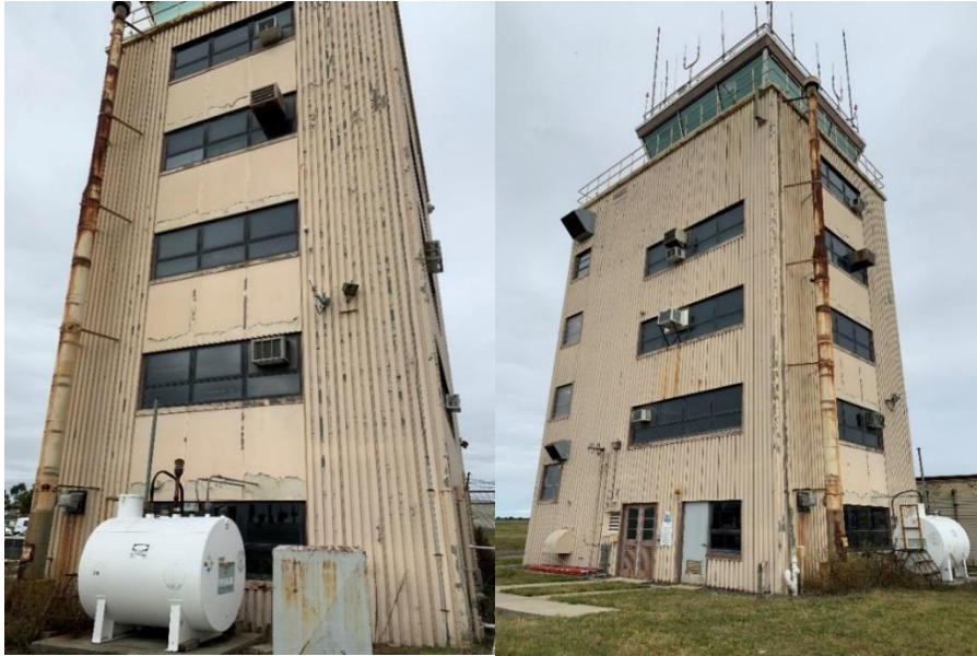
Figure I-4 Exterior Views of the Aging Existing ATCT
